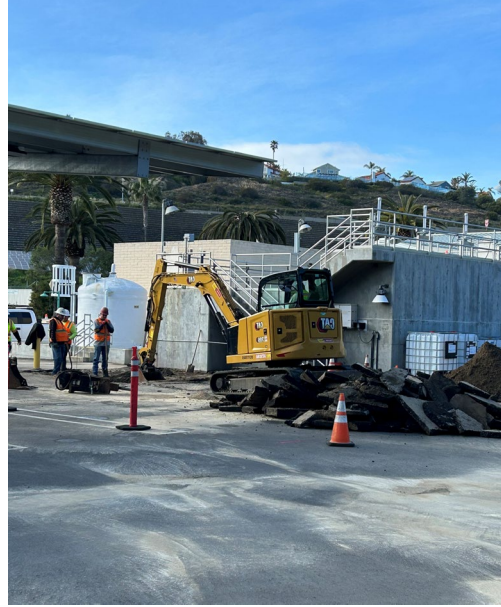
Photo 2 (March 8 th ) – Ahrens Mechanical mobilized and commenced excavation.
