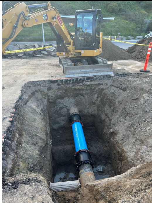
Photo 4 (March 8 th ) – Progress of pipe segment replacement.
