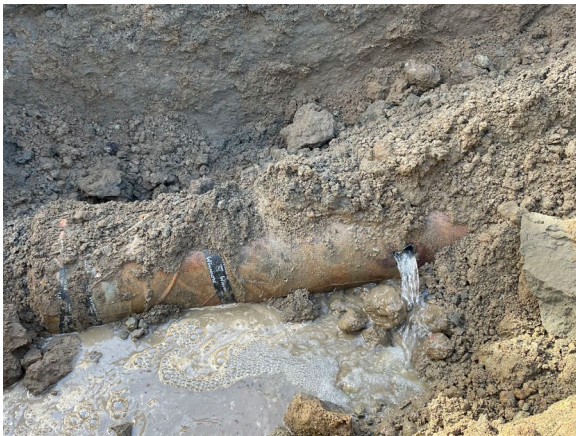
Photo 1 (March 6 th ) – Leak observed between chlorine contact basin and sand filter structure.
