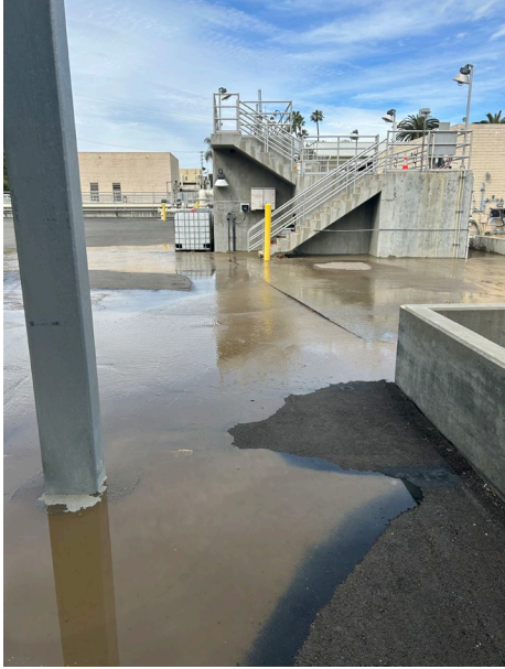
Photo 1 (March 6 th ) – Leak observed between chlorine contact basin and sand filter structure.
