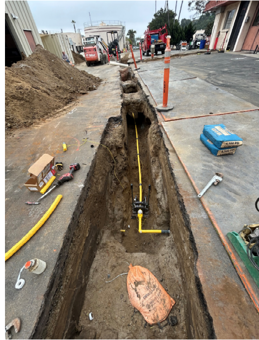
March 25, 2025 North end (looking south) of new 1-1/2" polyethylene pipe
