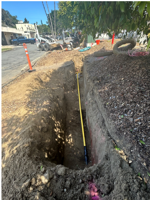
April 3, 2025 South end (looking north) of new 1-1/2" polyethylene pipe
