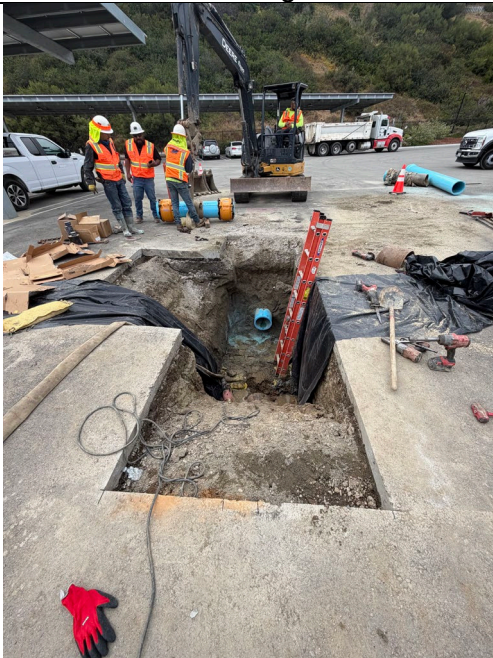
April 21, 2026 Pipe excavation
