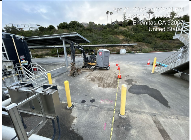
April 21, 2026 Excavation backfilled to grade
