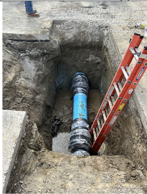
April 21, 2026 Installation of Replacement Pipe and Repair Couplings
