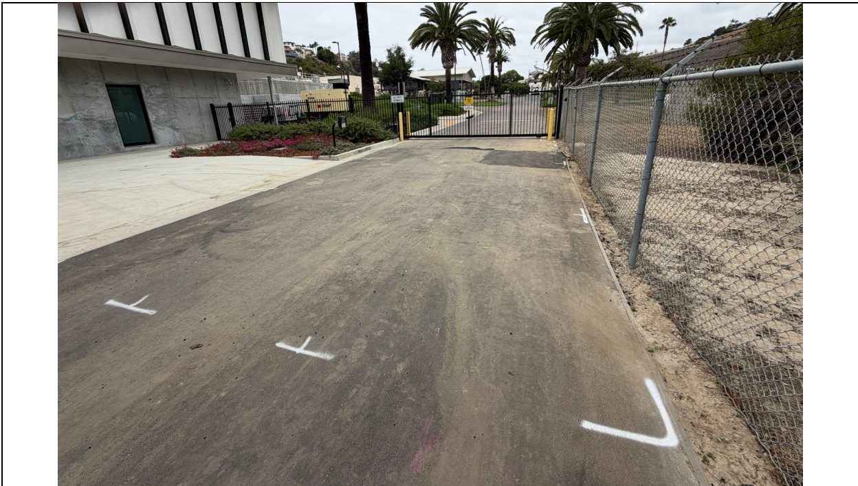
Excavation backfilled to grade with temporary asphalt Pavement repair area marked out with white paint
