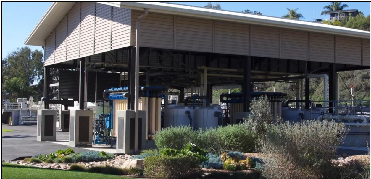
The San Elijo Water Reclamation Facility utilizes micro-filtration and reverse osmosis as part of the treatment process.
