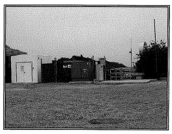
station would become inoperable if the station flooded. Also, this station has limited pumping redundancy and is not equipped with an emergency spill basin.
