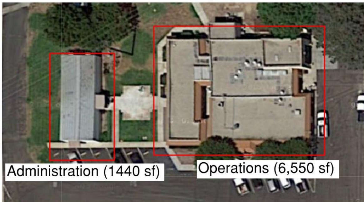
Figure 2. SEJPA Administration and Operations Buildings
