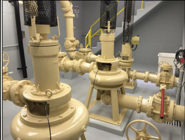
After Painting and Coating
