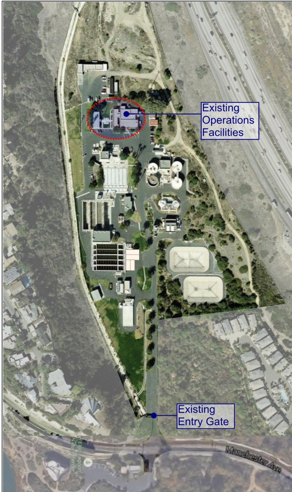
Exhibit A Existing Site
