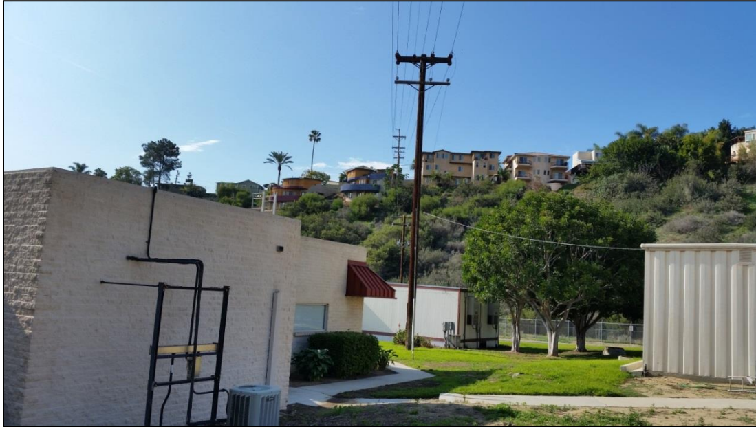
Photo 2 Buildings Under Power Lines
