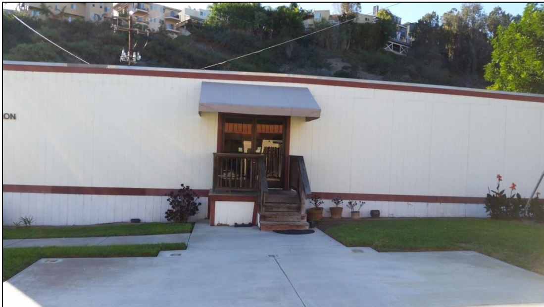
Photo 3 Non-Accessible Portable Trailer Building Entry
