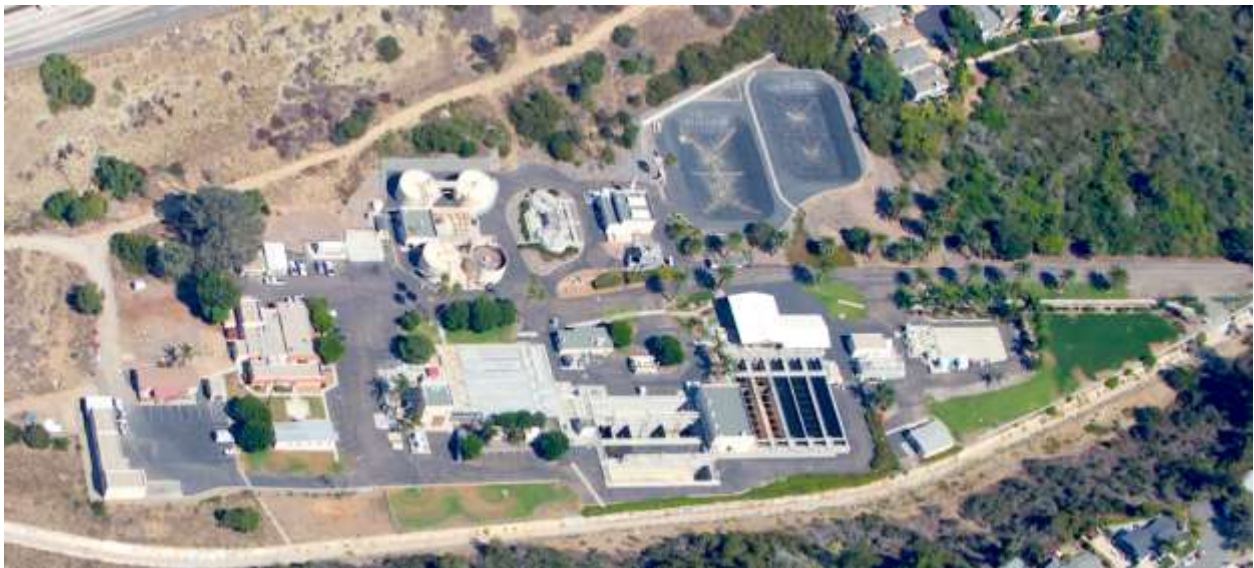
Aerial View of San Elijo Water Campus
