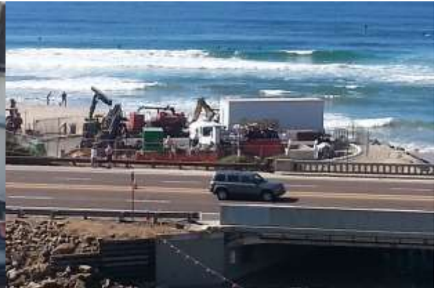
Coast Pump Station Construction
