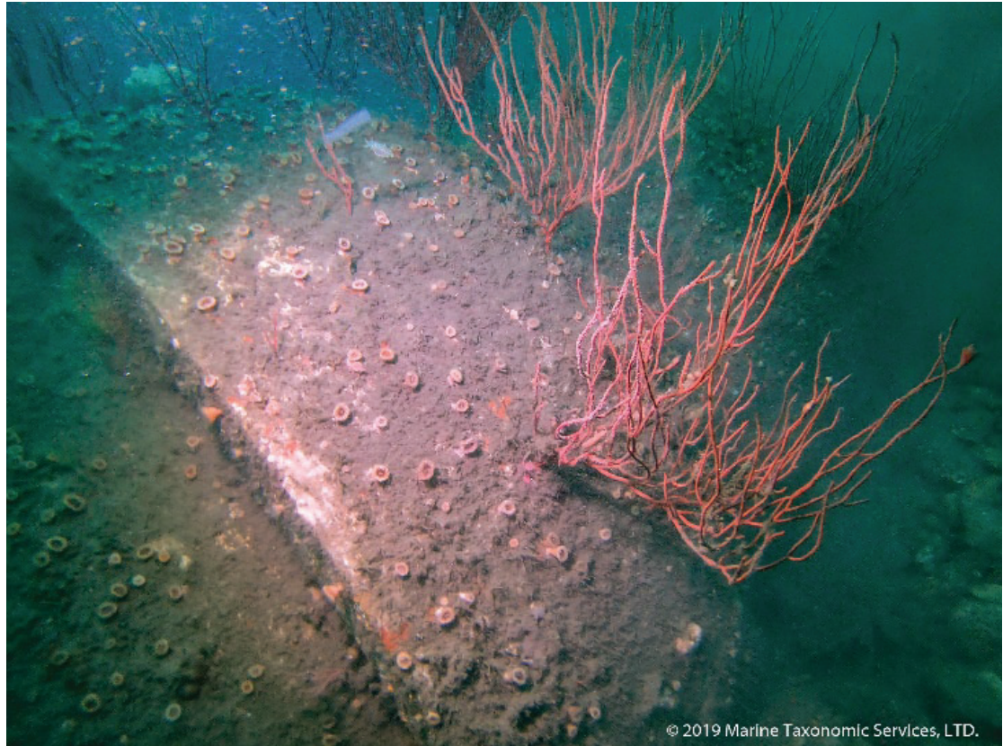
Figure 4 Marine Growth on Joint and Piping
