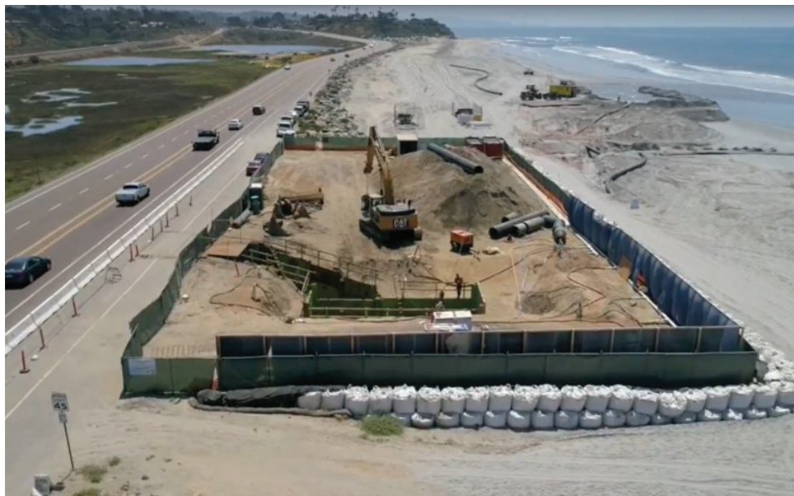
Figure 2 Land Outfall Launch Site
